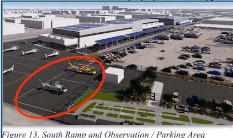
Figure 13. South Ramp and Observation / Parking Area
